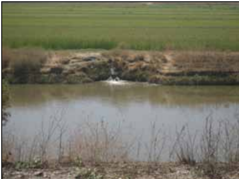
Field drainage entering Colusa Basin Drain (Photo: Colusa Glenn Subwatershed Program)
