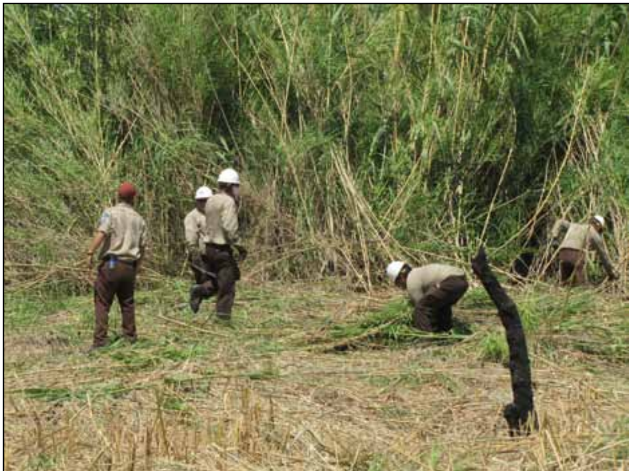
A work crew takes on the daunting task of removing an Arundo donax infestation in Glenn County (Photo: Glenn County RCD)
