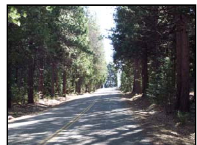
Phillips Road Fuelbreak: Note dense brush and trees up to edge of the road
