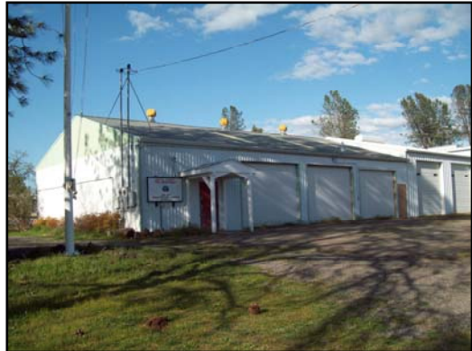
Oak Run Volunteer Fire Department Station
