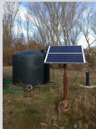
Solar-powered Lift Pump, Tanks & Troughs
