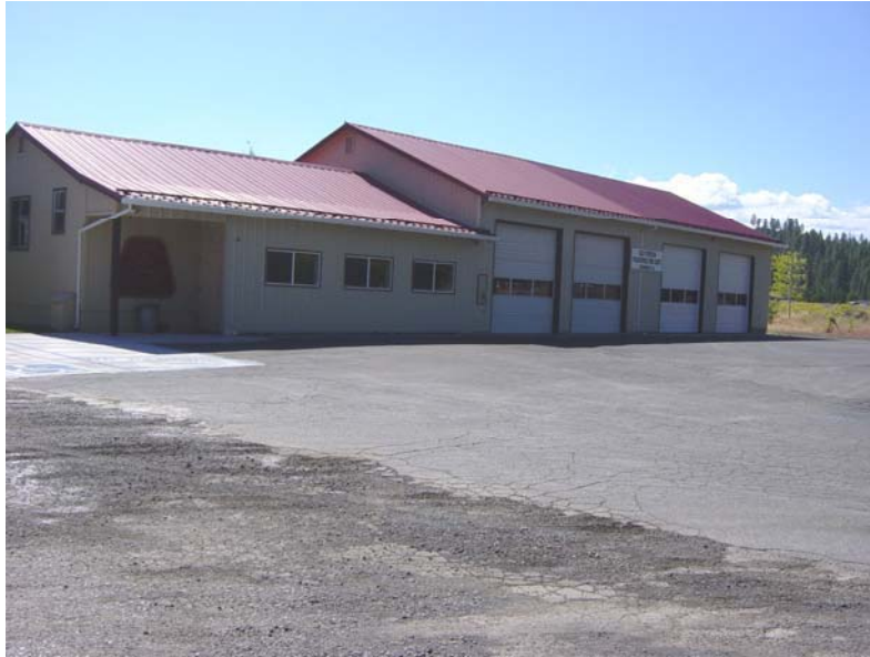
OLD STATION VOLUNTEER FIREHOUSE
