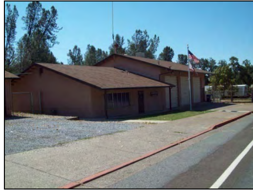
SLFPD Fire Station
