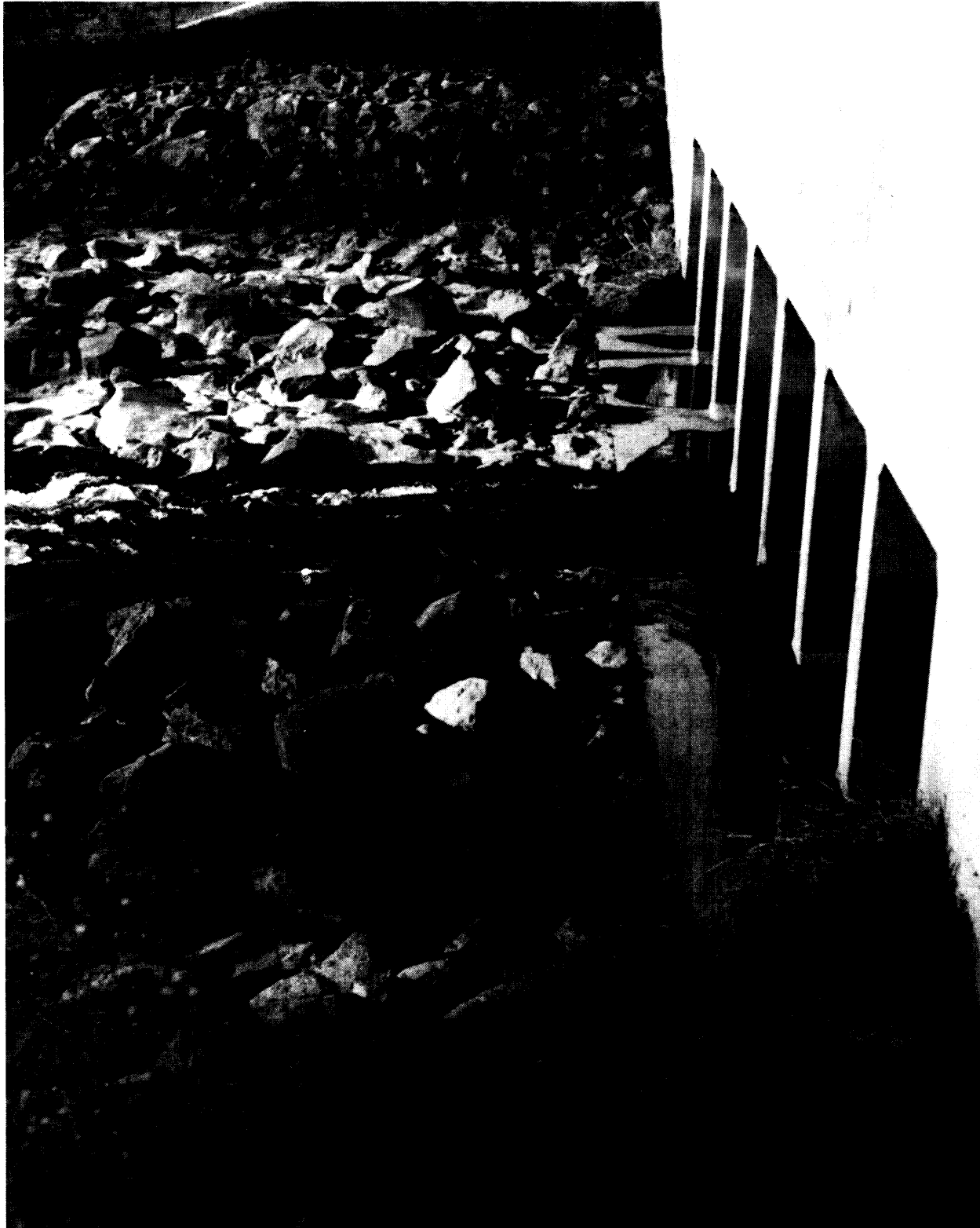
This culvert dam at Five Mile Recreation Area could provide flow management in Lindo Channel, although fish passage should be improved just below the dam.
