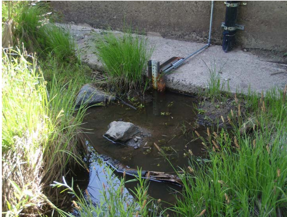
Low flow recording equipment at Taylorsville Bridge.
