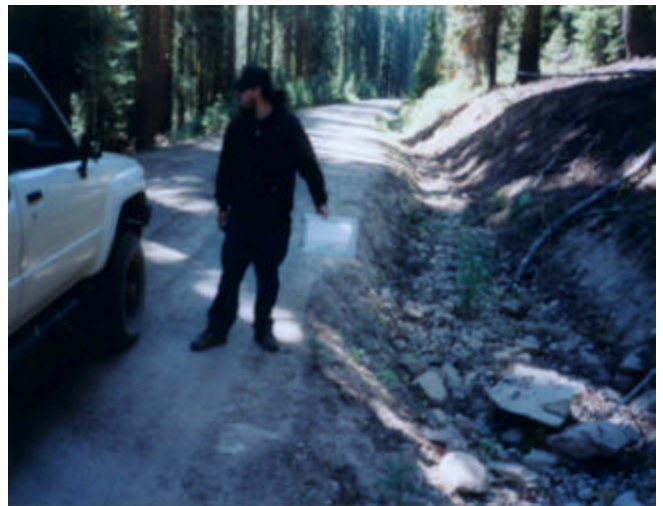
Road erosion and stream delivery survey.
