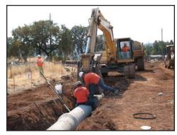
Construction workers installing storm drain system
