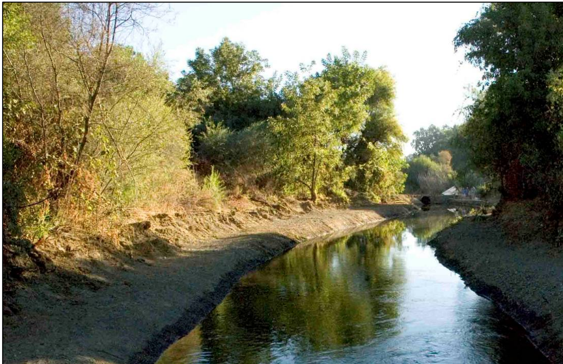
Putah Creek water flows clear within a day following the opening of the realigned creek channel. Removal of the arundo-stabilized gravel delta at the mouth of Dry Creek and the configuration of new channel are intended to protect the south bank of Putah Creek and enable gravel to move further downstream, providing much-needed spawning habitat for Chinook salmon and other anadromous fish.
