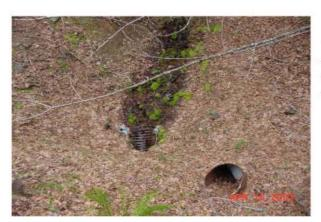
The photo to the left shows the inlet of the culvert. You can notice a piece of the inlet in the lower right hand corner that was cut off and discarded.
