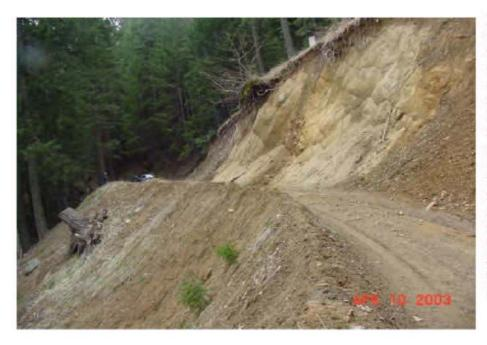
Photo shows the mass wasting at the cut bank that causes regular road failure. Routine maintenance to insure that the mass wasting does not affect road drainage is imperative to reduce the likelihood of a large failure.
