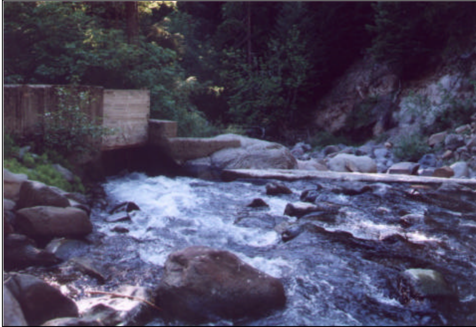
Photo 5-3: Kilarc Diversion on Old Cow Creek.
