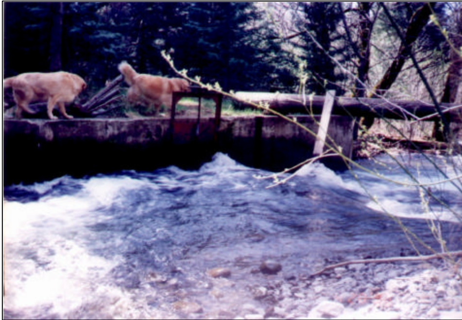
Photo 5-2: Mill Diversion on Clover Creek
