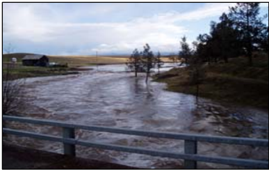
Beaver Creek at Pittville. Pit River tributary at flood stage in January 2006. Degraded watershed conditions contribute to peak runoff from storm events causing flood damage, channel erosion, and property loss.
