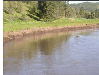
Channel erosion on Pit River at Shaw Ranch.
