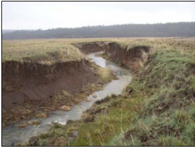
Channel entrenchment and erosion on Rush Creek
