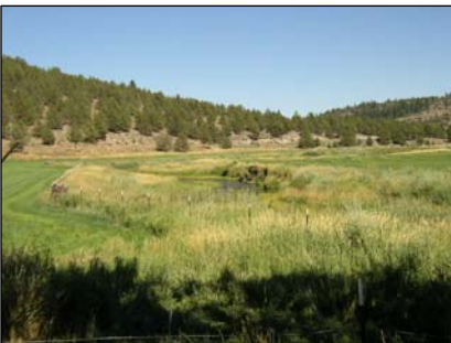
Pit River channel stabilization near Canby (Bushy Ranch) using rock, willow plantings, juniper rootwads, and livestock fencing.
