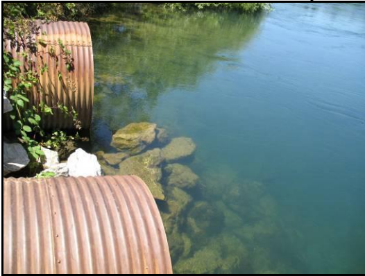
Culvert outflow at the mouth of Jenny Creek.
