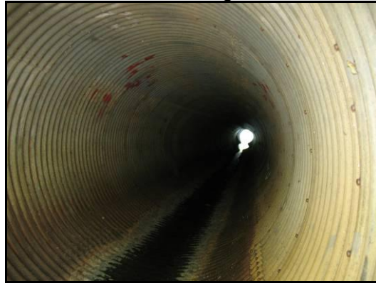
View of culvert looking downstream.
