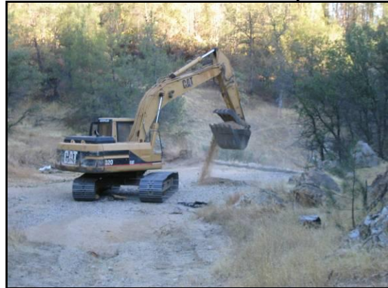
Sediment Removal at Swasey Dam.
