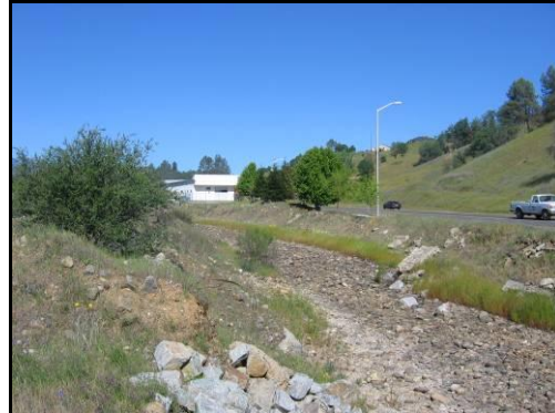
Alternate view of Canyon Creek.
